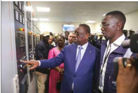
Above: The 120 MW Malicounda power plant, built under a public-private partnership (PPP), inaugurated by President Macky Sall.
